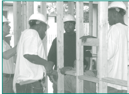
A St. Leonard's Ministries work crew begins renovating a building.
